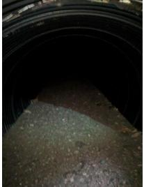
It is more than likely that the invert is severely deteriorated beneath the sedimentation
