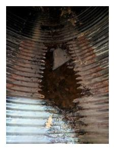
*Segment 6* - No corrosion, deformation, or joint damage was noted; however, severe invert deterioration was noted along most of the CMP sections of pipe. Some isolated areas of debris deposits were noted; asphalt.
