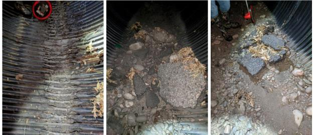
It is more than likely that the invert is severely deteriorated beneath the sedimentation
